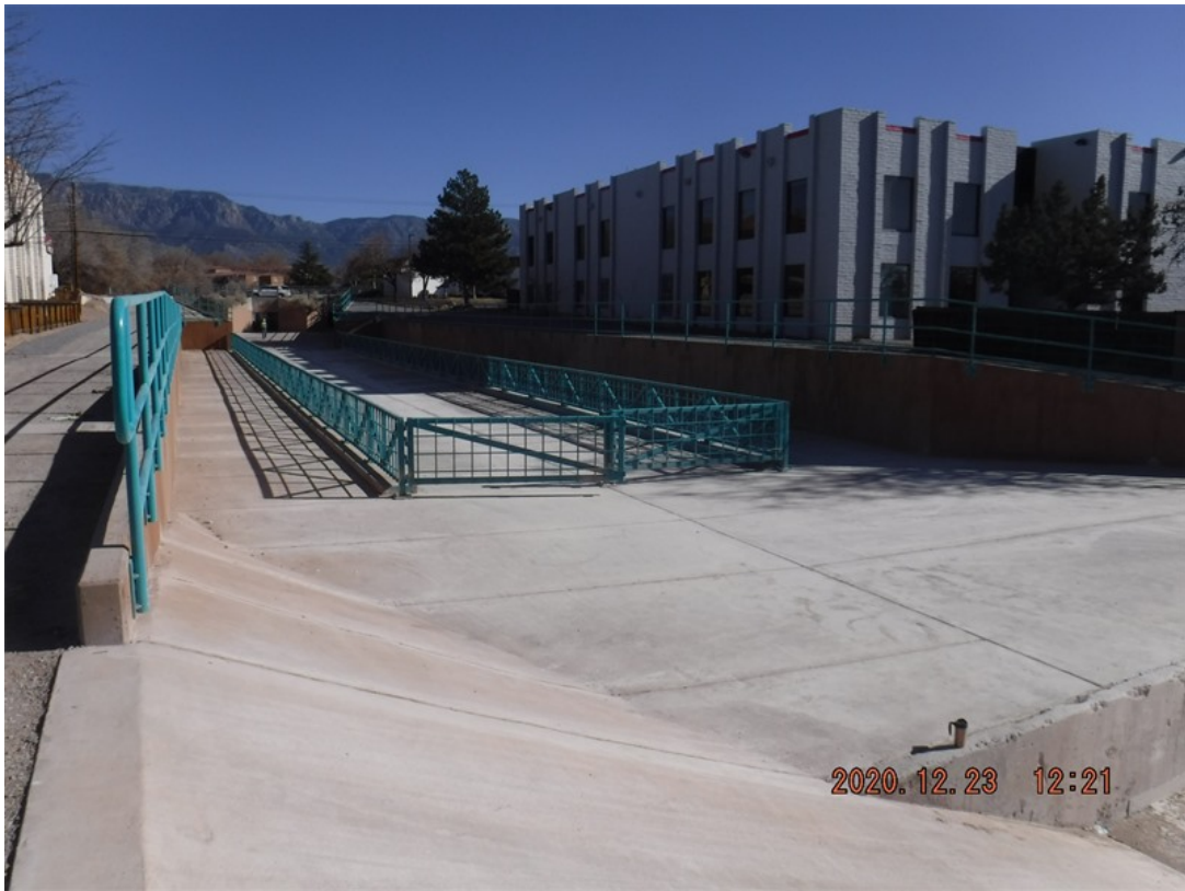
Photo facing east, Car - 1: Channel cleaned up by Contractor AUI.
