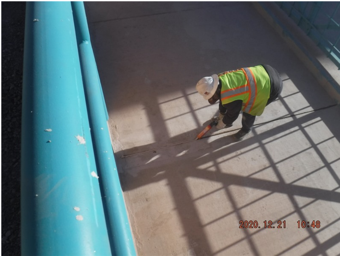
Photo facing southeast, Car - 1: Contractor AUI applying sealant to control joints.
