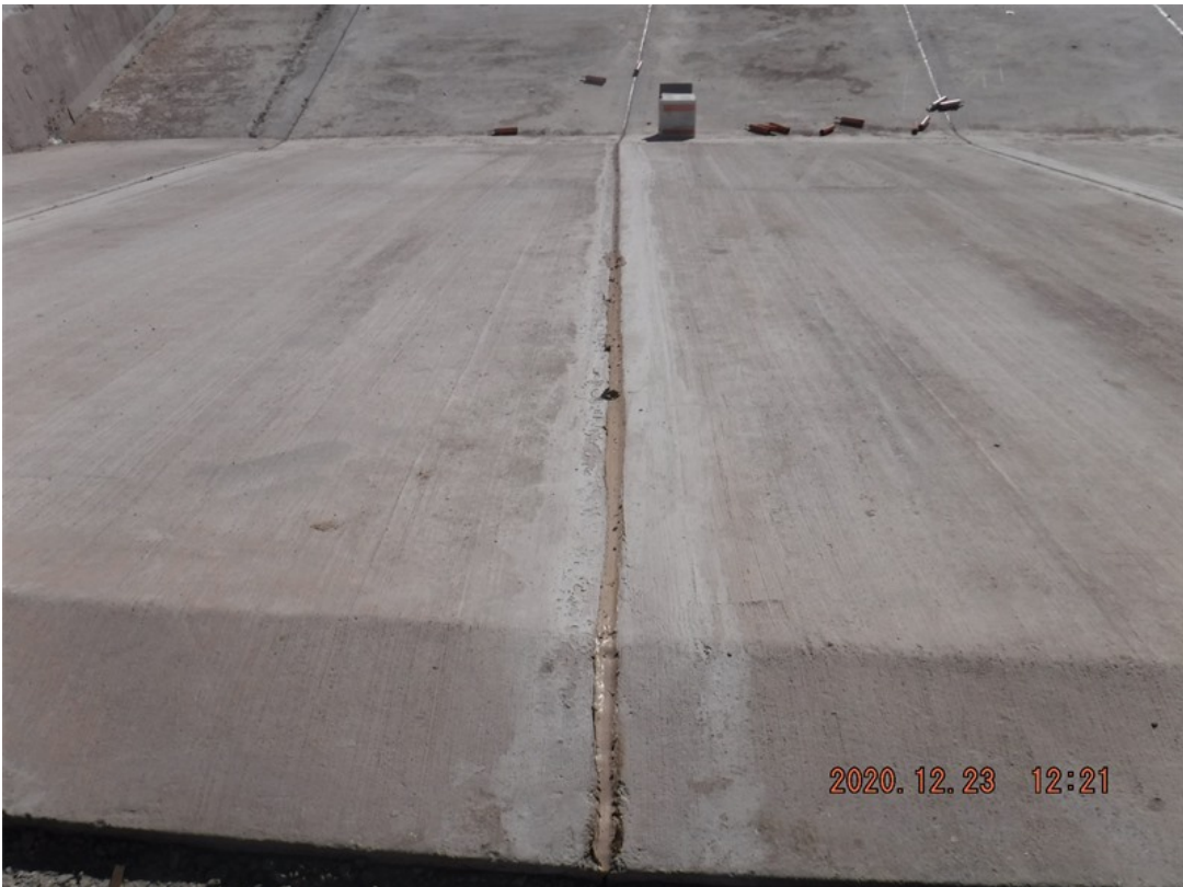
Photo facing south, Car - 1: Construction joint sealed by Contractor AUI.
