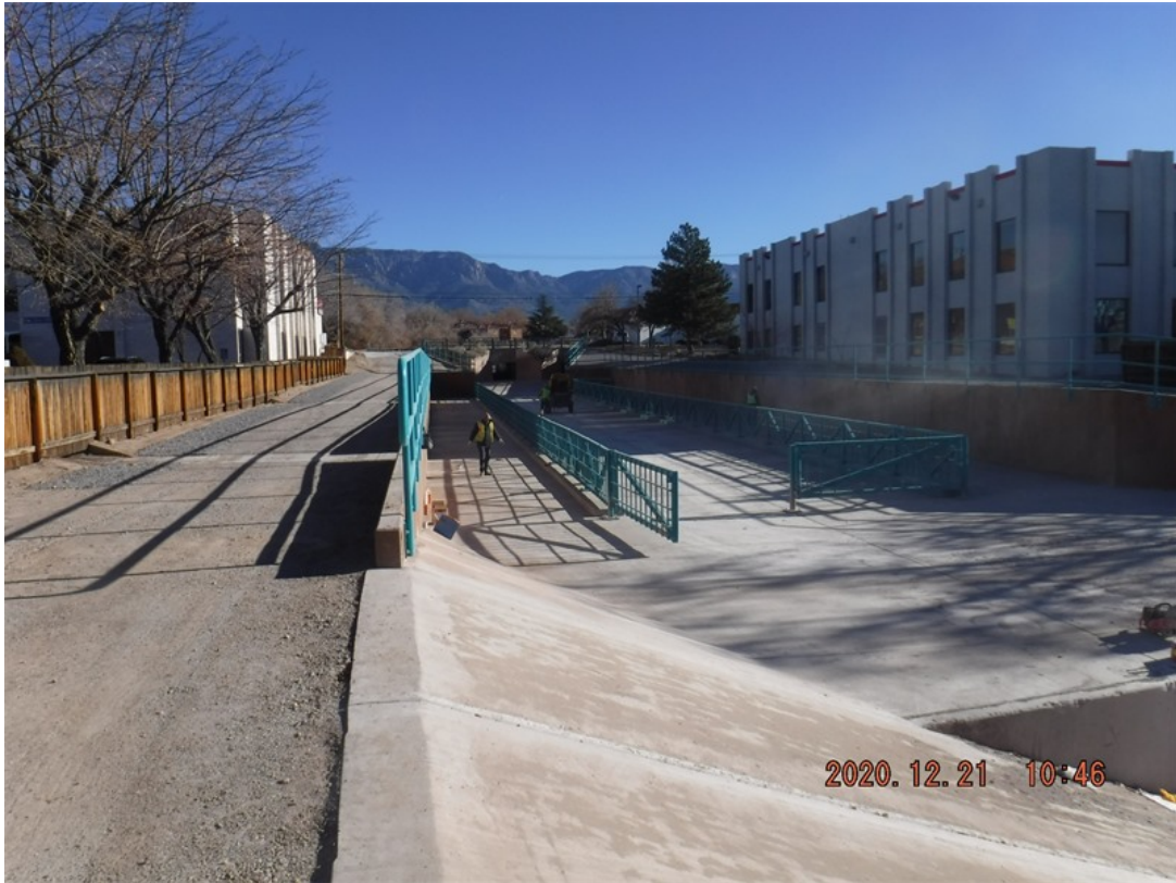
Photo facing east, Car - 1: Contractor AUI preparing to seal control joints.
