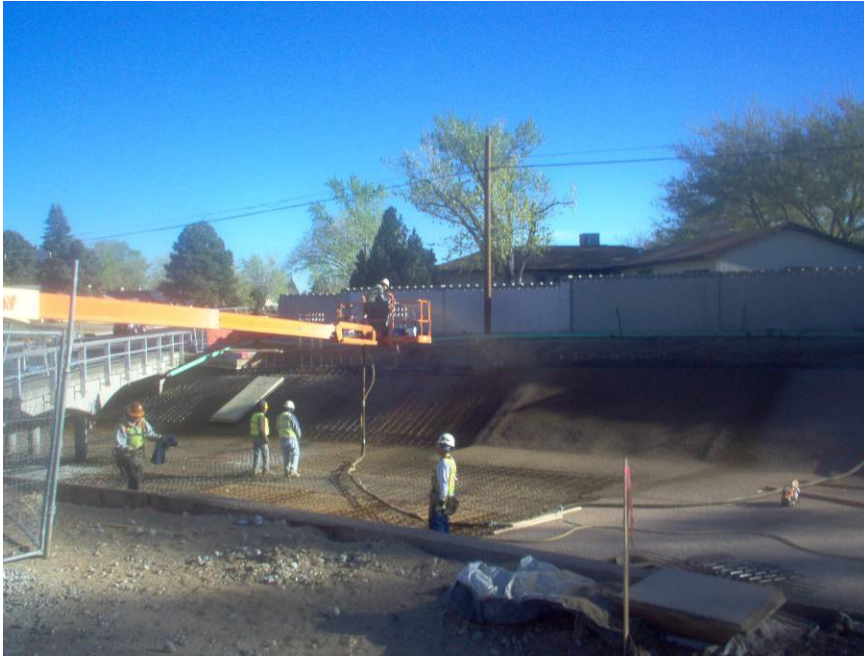
Superior placing shotcrete east of the San Pedro Bridge.
