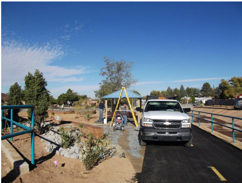
COA Parks painting the existing shade structure.
