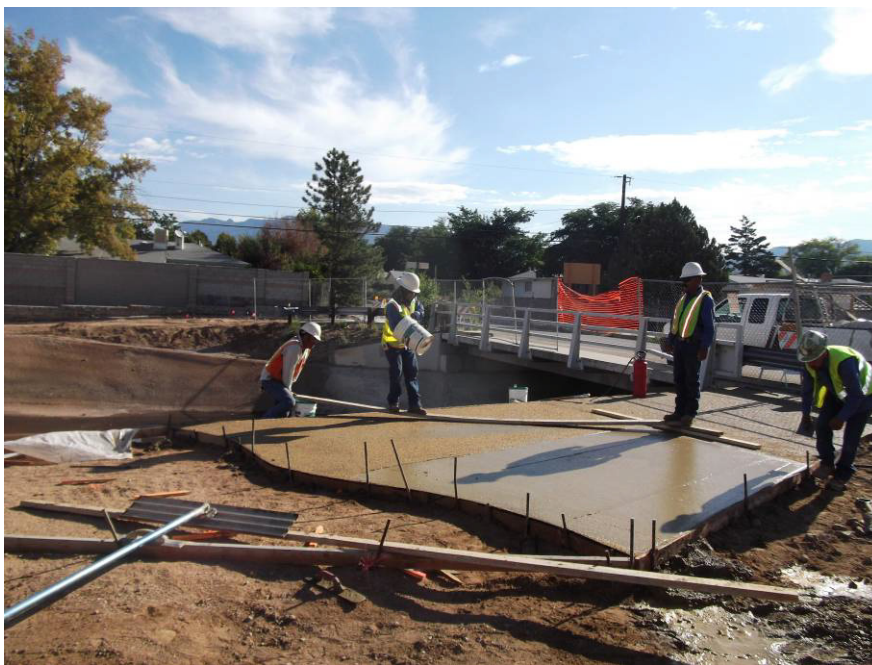
HO placing exposed aggregate concrete on plaza NO. 7.
