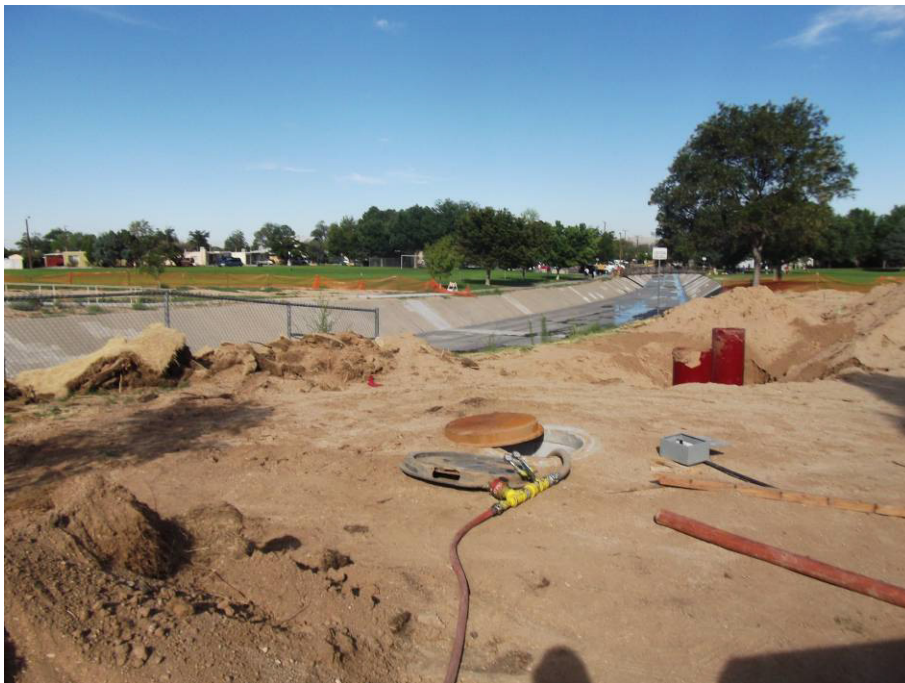
Air testing at MH Sta 4+49 by RMCI
