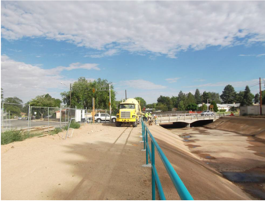
RMCI pouring sill walls at San Pedro
