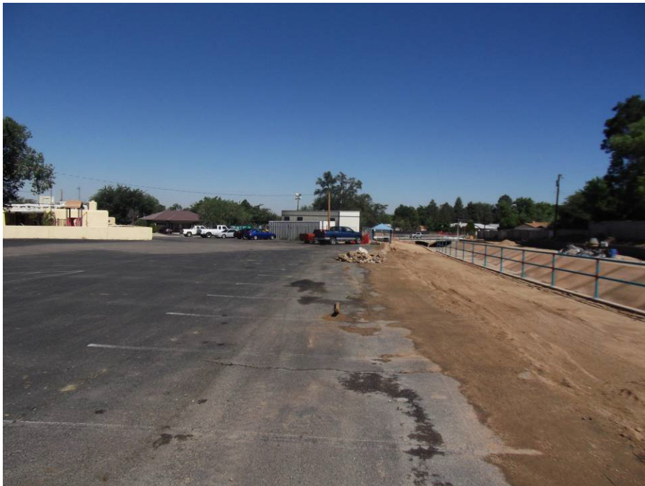
Main irrigation line has been placed here. There is some of the debris pulled from the trench.
