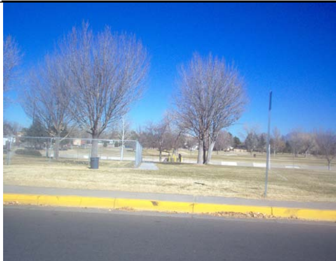
Alignment for placement of permanent wheelchair ramp.
