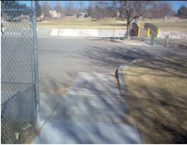
Existing Wheelchair ramp to widen
